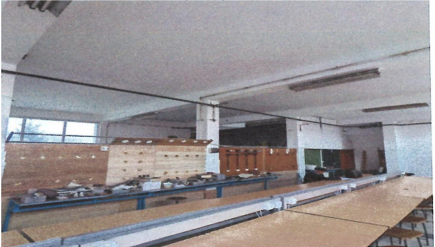
Photo 5 – Photo from Gf Electric Workshop. One can see the structure made of concrete frames of the building block
