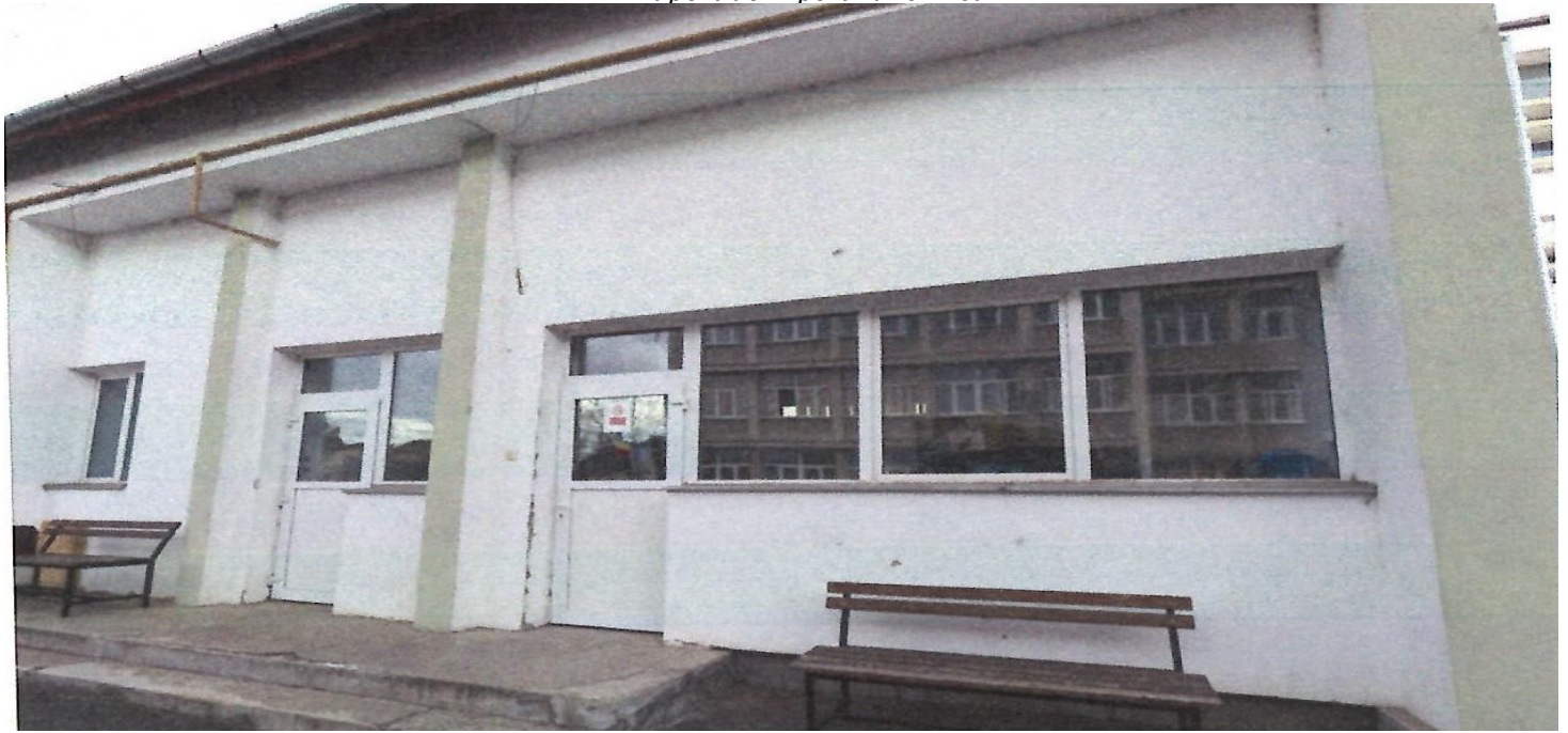
Photo 9 – Entrance to the Electric Workshop
