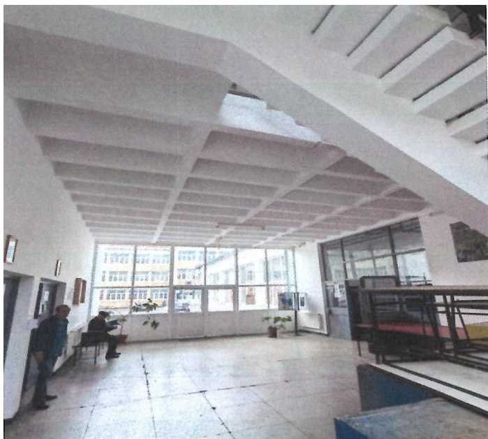
Photo 4 – Photo from the main hall, one can see the ribbed floor and staircase
