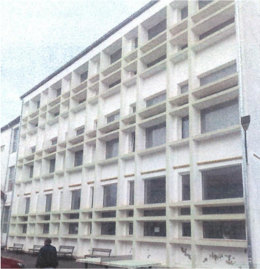
Photo 1 – Main entrance – one can see the brice-soleils from the laboratory level
