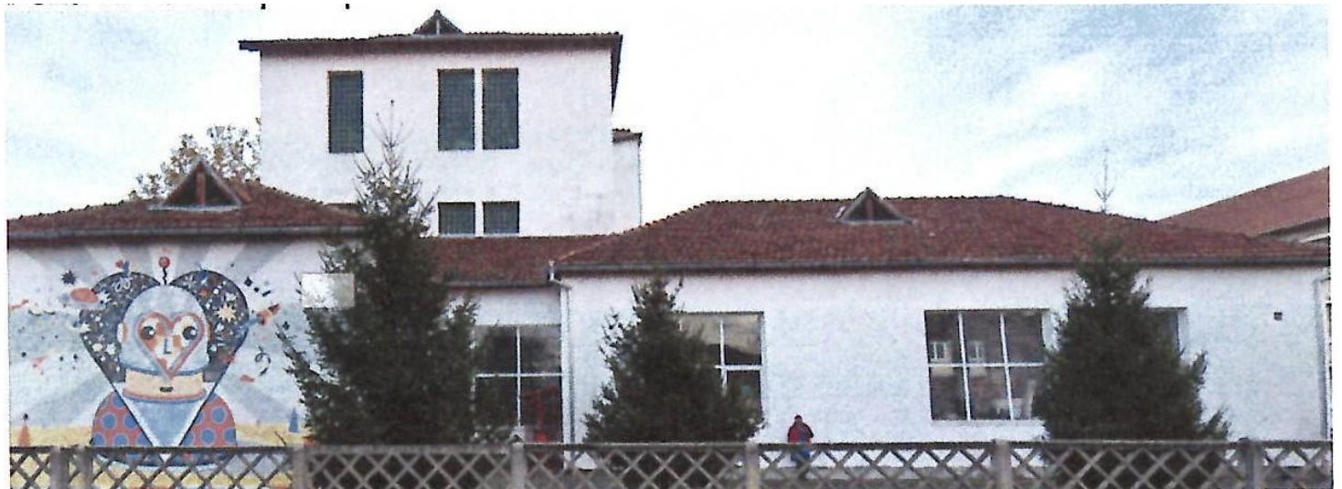
Photo 2 – Left side entrance from Vasile Aaron street. In the foreground one can see the block Gf Electric Workshop, to the left the Garage and in the secondary plan, the block Gf+2F
