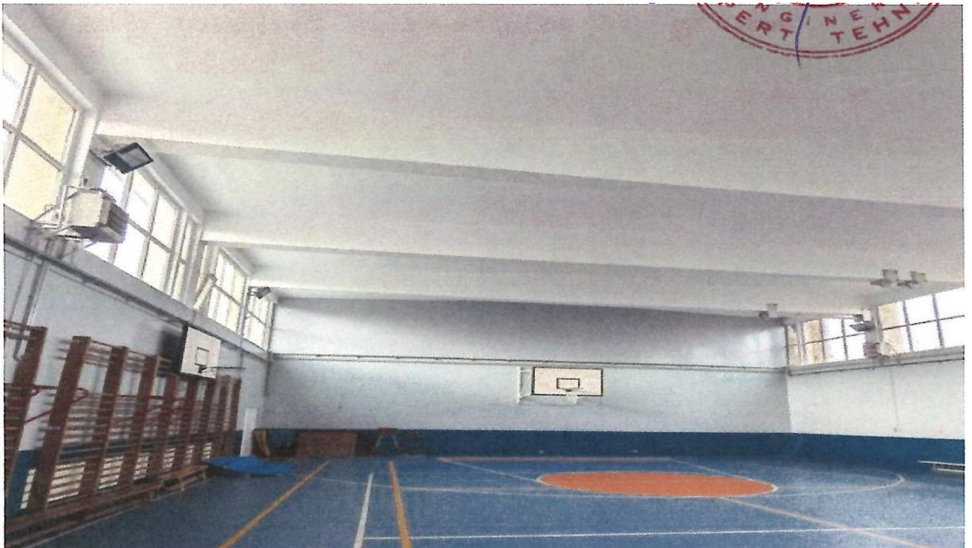
Photo 6 – Photo from inside the gym hall, one can see the beams with variable height, the main pillars and the side wall made of masonry
