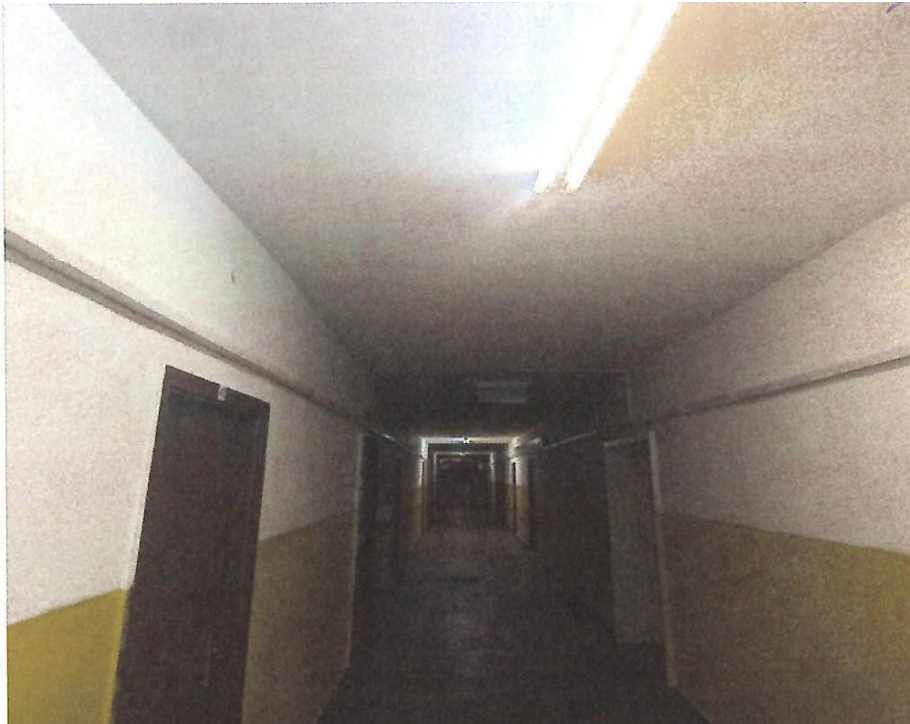
Photo 8 – Central hall in the student dormitory building
