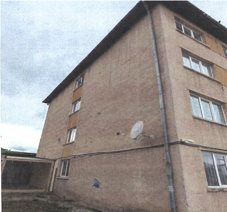
Photo 4 - Side entrance towards Semaforului street
