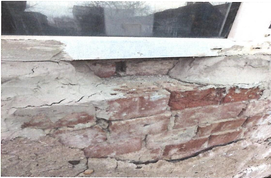
Photo 10 – Areas with the plaster fallen and with apparent bricks
