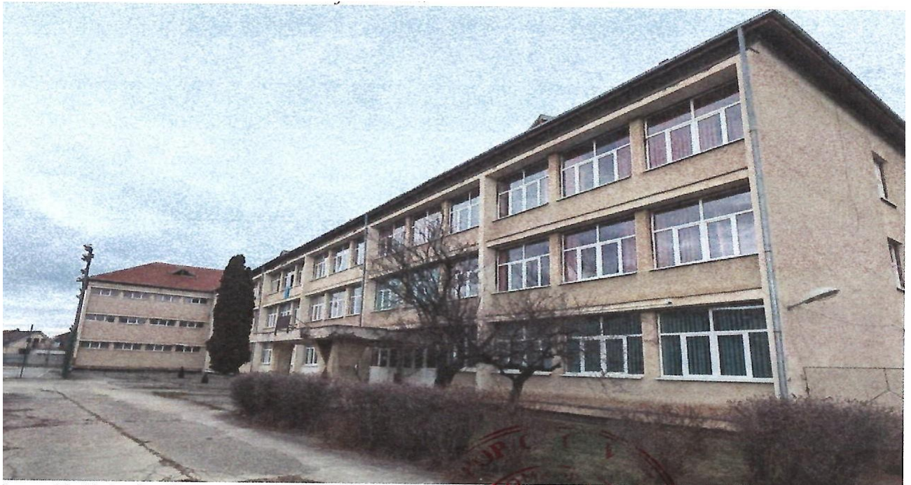
Photo 2 – Entrance from Electricienilor street
