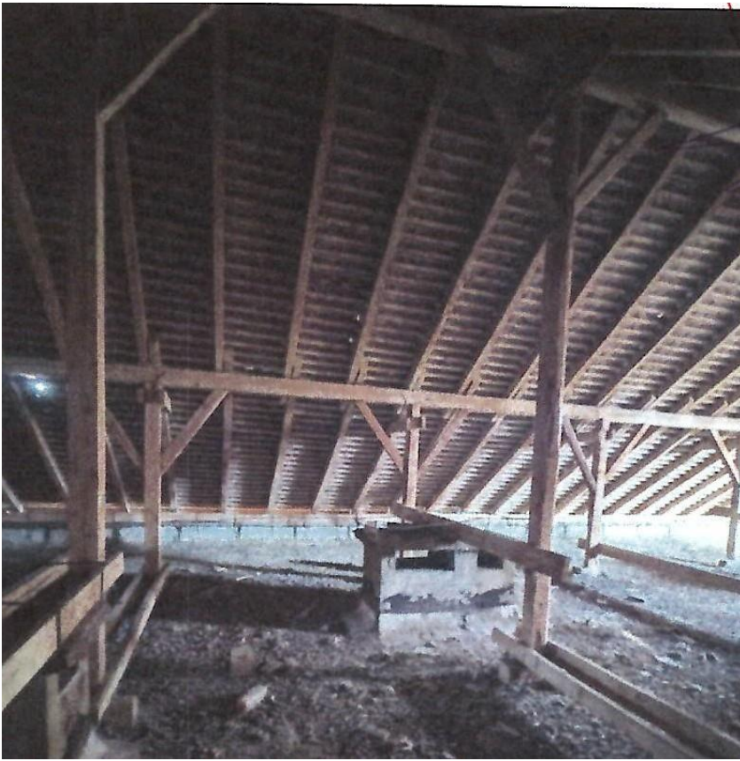
Photo 9 - Photo with the additional framework structure
