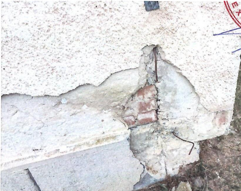
Photo 7 - one can see the corner reinforced concrete column
