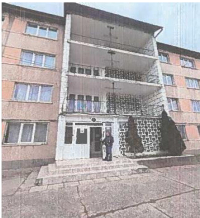
Photo 1 – Main entrance, one can see the main access in the building
