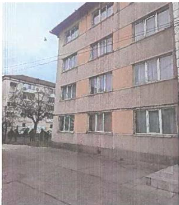
Photo 2 – Left side entrance
