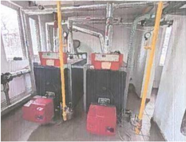
Photo 4. Photo of the thermal plant, one can see the two boilers providing heat and the boiler for storing the hot running water
