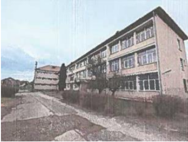
Photo 1 – Entrance from Electricienilor street
